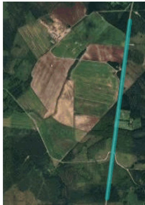
Figure 12 –Satellite image of the solar power plant
